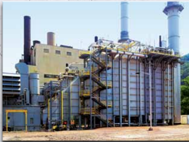
Modular designed field-erected Utility Combined Cycle HRSG.
