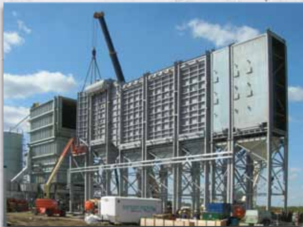
Erosive and corrosive resistant solid fuel (coal-fired) HRSG.
