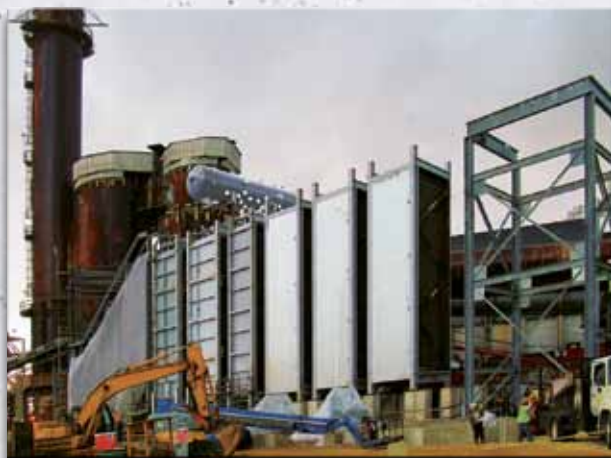
Waste heat recovery project, expected to produce upwards of 40 megawatts. Capacities: 450K PPH, 1,300 PSIG and 900 Degrees.
