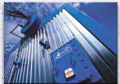
Over-size entryway doors allow easy access.
