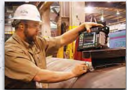
Excellence is a top priority; over 100 checkpoints are in place for quality control, tracked and managed by ITP (Inspection Test Plan).
